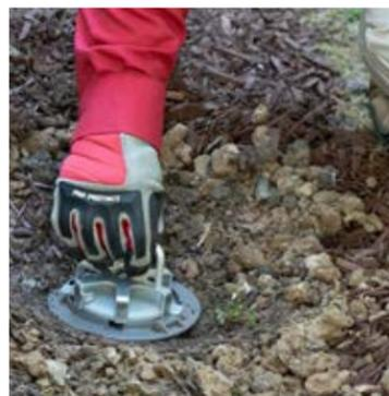
4. Using the spider tool, secure lid into place
