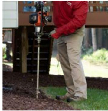
1. Auger/drill holes for the Encircle Stations. Drill holes 1 inch deeper than the height of the station to allow for drainage
