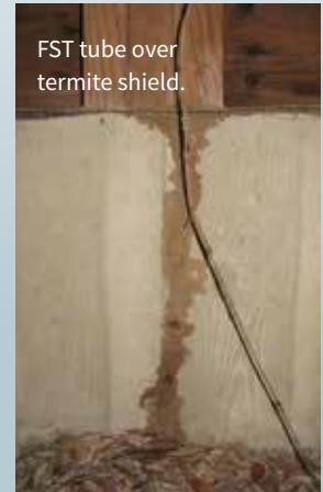
FST tube over termite shield.
