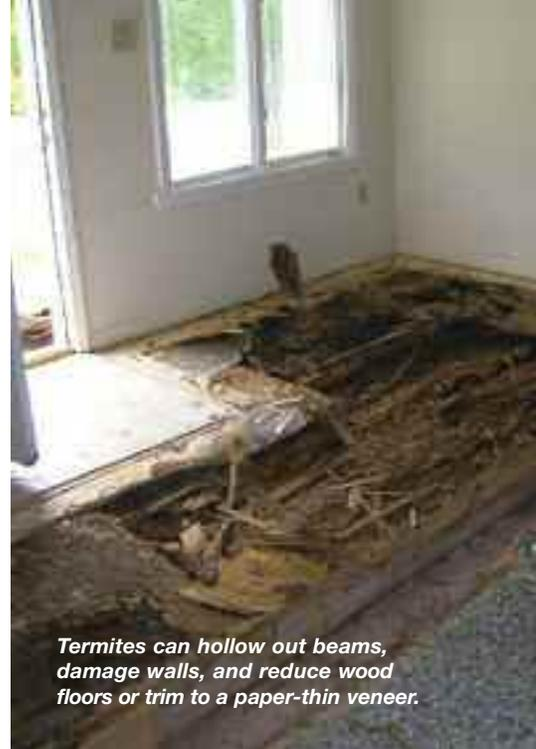
**Termites can hollow out beams, damage walls, and reduce wood floors or trim to a paper-thin veneer.**
