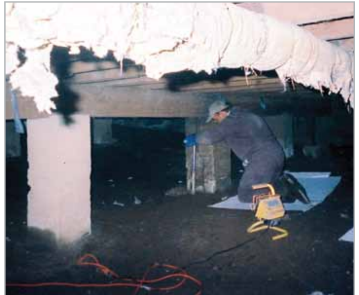
Miller and crew installed 40 baited ATBS stations under the structure. Within the first 30 days Miller had hits on 22 of the 40 stations.
